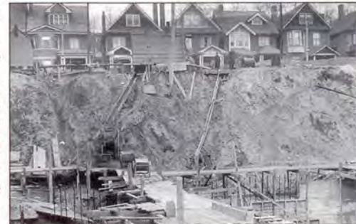
DIG IT: Building the sewage storage tank in High Park in 1914.
