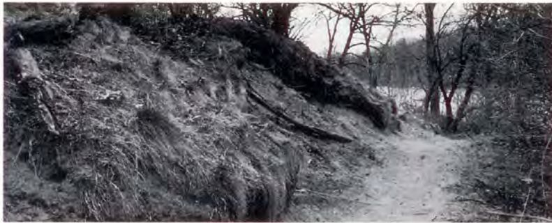
Trails cut into the slopes just east of Grenadier Pond in High Park have caused devastating erosion.
